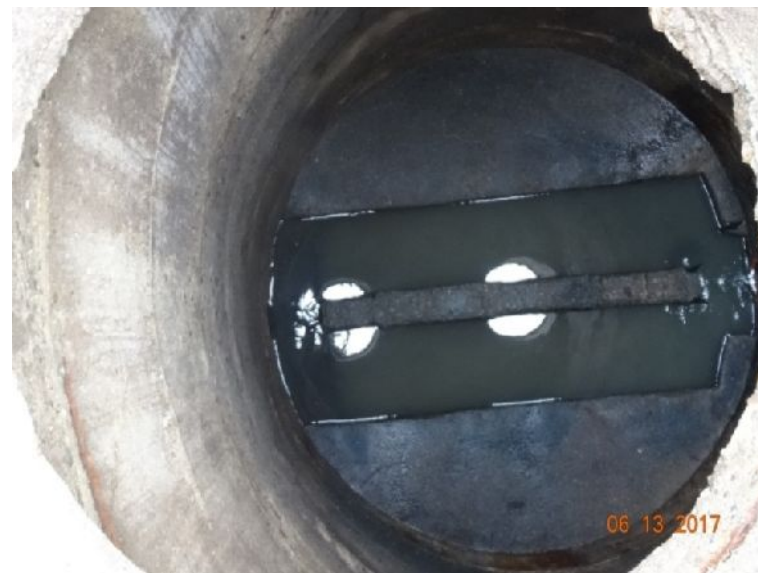
Figura 38: ETE Nova Sepetiba II (Vistoria DIS/GFT)
